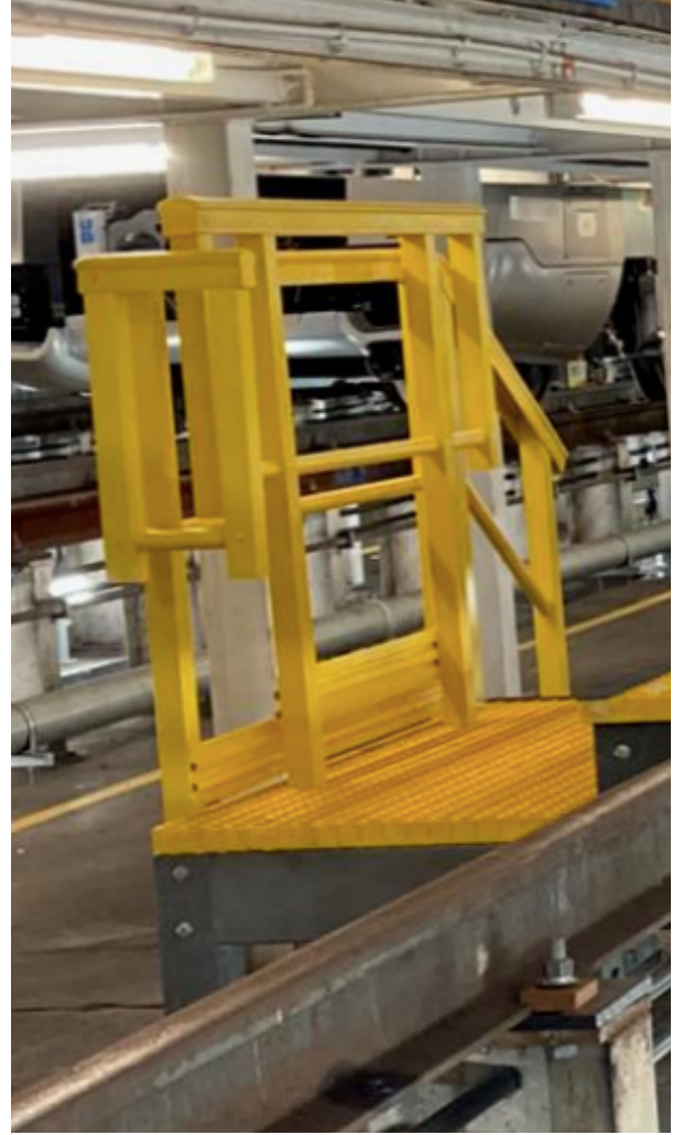
Mid-rail coupler work platform mid-handrail storage location
